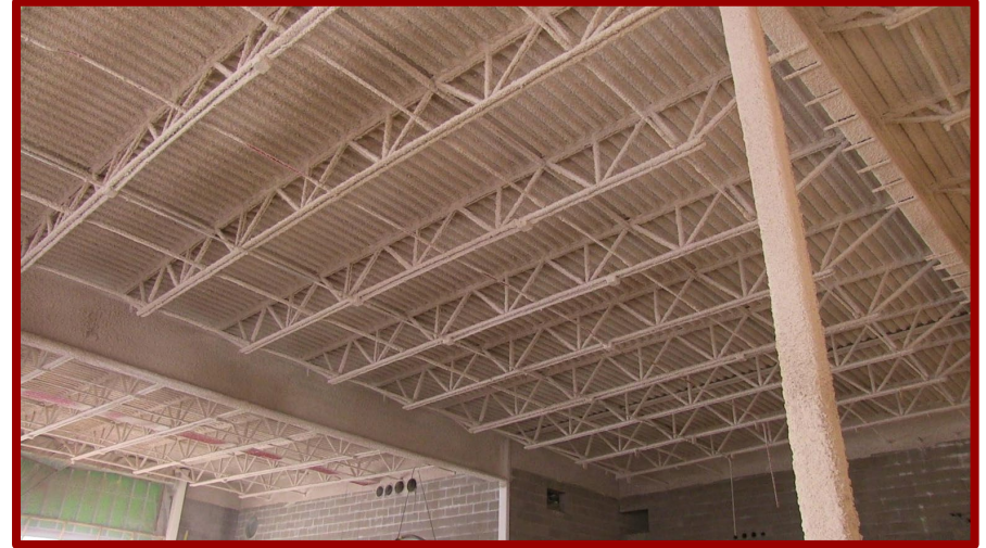
Fireproofing in cafeteria
